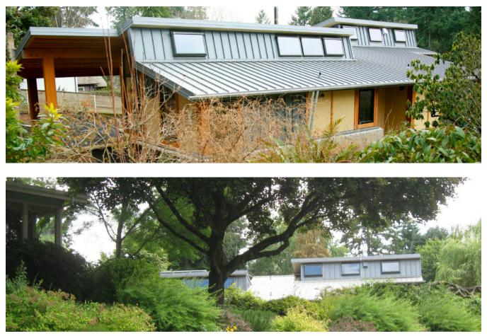
The clients for this project were interested in exploring and integrating a number of environmental responses into their new home. The house form allows for natural ventilation and passive solar heating, supported by a hydronic heating system. The house is free of fossil fuels, has a metered solar electric system, and is pre-plumbed for solar hot water. A high efficiency air-to-water heat pump provides for the hydronics and domestic hot water.
